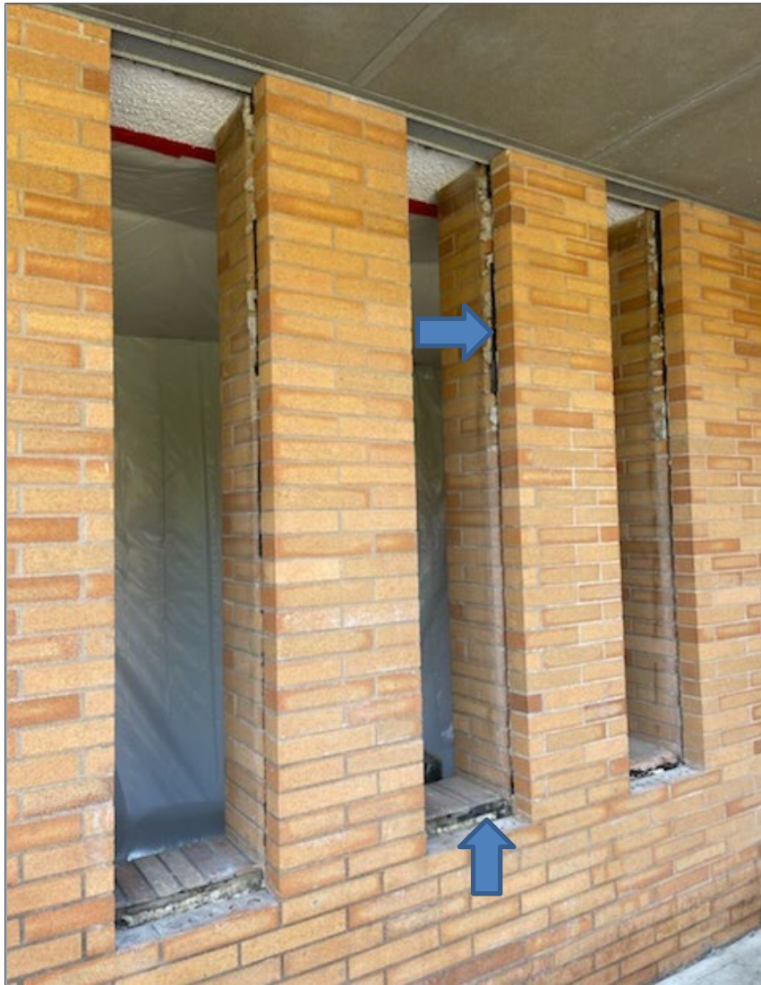
Building C - Chapel Vapor barrier behind brick façade; vapor barrier is suspect ACM.
